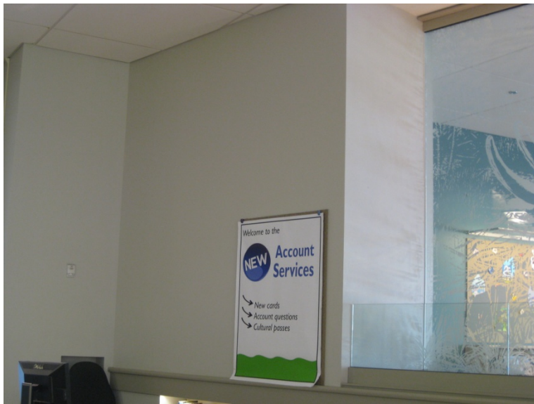
Figure 6: West wall alongside Mastodon skeleton
