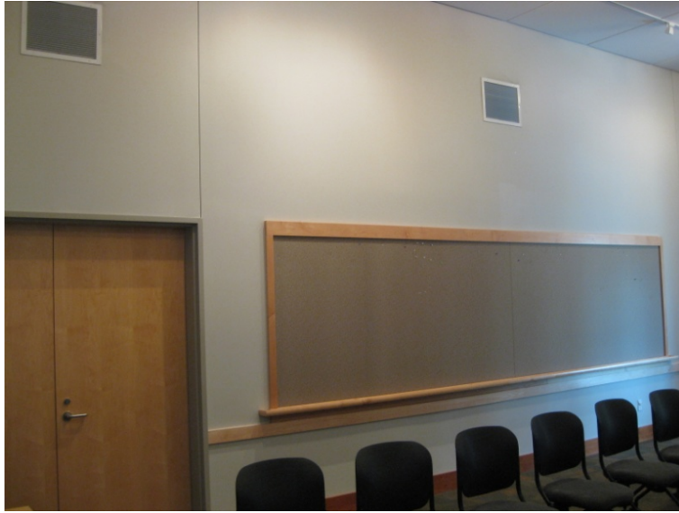
Figure 3: Community Room – north wall
