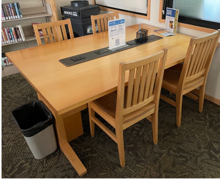
Wood table top with table top plug ins (2 not hardwire, standard plug; 1 hardwired, will be disconnected)
