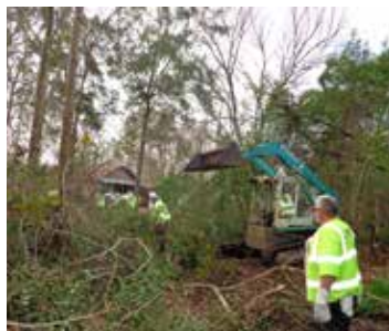
Bulldozers clear debris.
