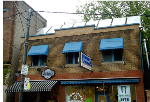
Design guidelines can address where solar panels should be placed on a historic commercial building. In this instance, panels should have been placed to rear where they cannot be seen at street level.
