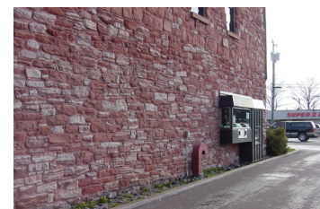
Thick masonry walls were common for most historic commercial buildings before the advent of air conditioning and electrically powered HVAC systems
