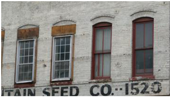
Historic windows and doorways should be kept in good condition and not removed. All doorways and windows should be checked for air infiltration and weatherstripped and sealed accordingly.
