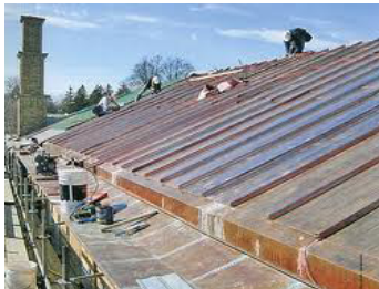
Maintaining original roofing materials, such as standing seam copper (above) should be a priority. If replacement is necessary, metal roofs can be ordered with “cool roof” reflective coatings.
